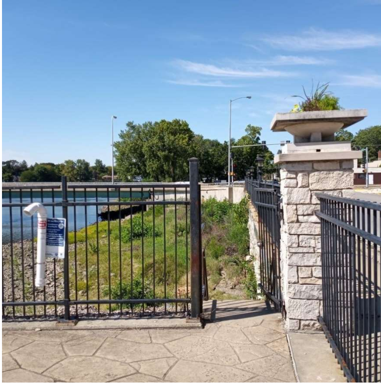
Non-Project Tailrace Fishing and Viewing Platform at the North Abutment of Dam, Looking West
