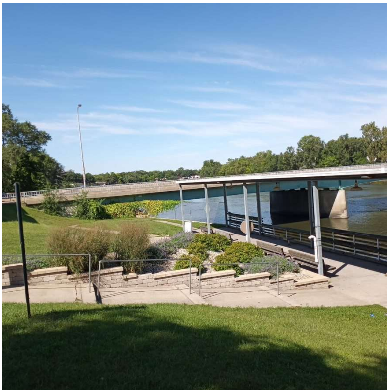
Project Tailrace Fishing and Viewing Area, Looking West
