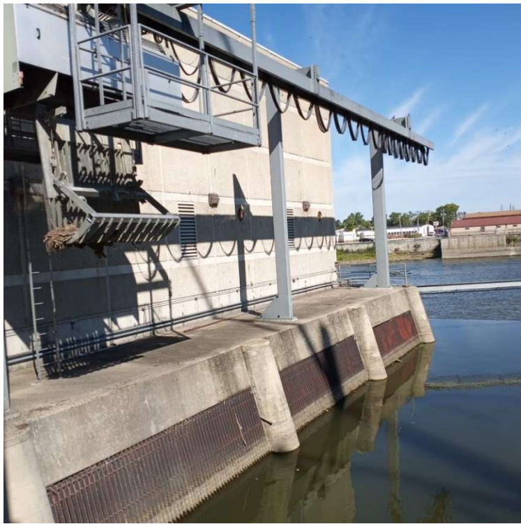
Powerhouse Intake, Trashracks, and Trashrake, Looking North
