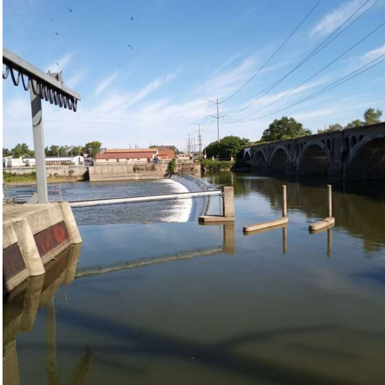
Kankakee Dam and Powerhouse Intake Channel, Looking North
